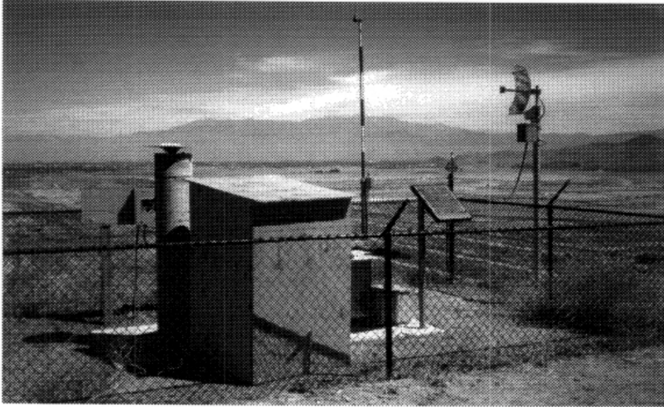
Figure 3. GPS CORS station at the east end
