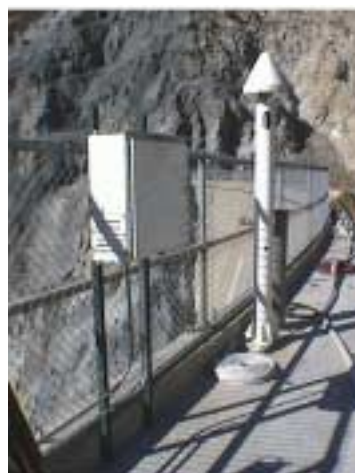
Figure 2 GPS installation on Pacoima at location DAM 2 (from Hudnut and Behr 1998)
