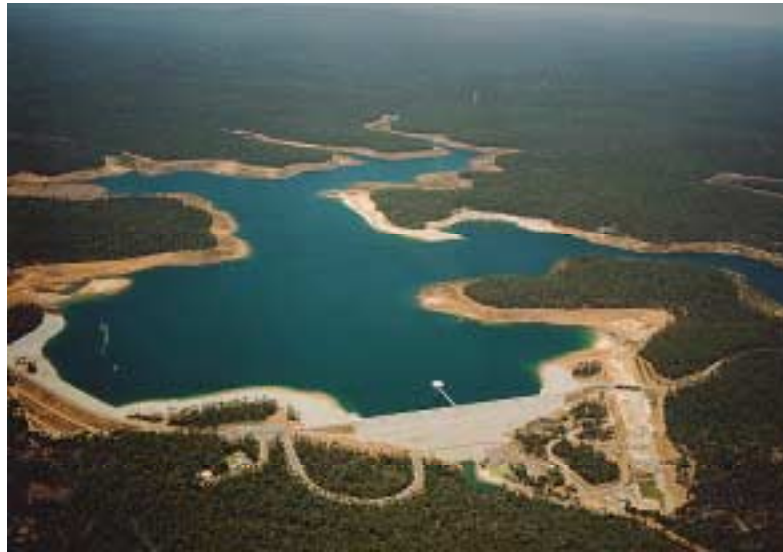
Figure 4 Aerial view of North Dandalup Dam, Western Australia
