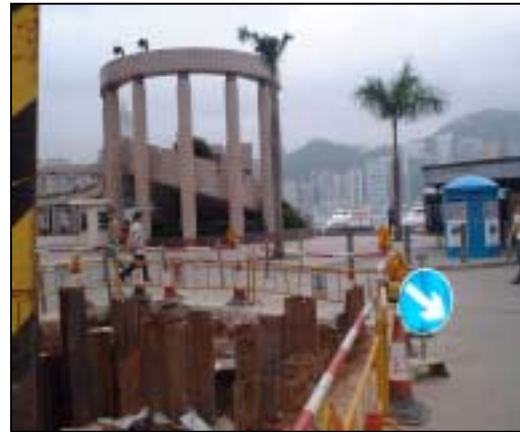
Figure 1. The Colonnade at Star Ferry with the trench in the foreground
